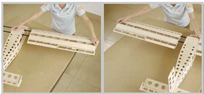
10.3 Install wing tubes and wings.
